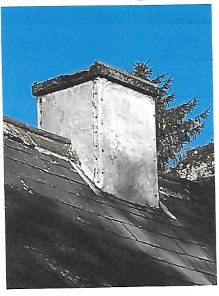
There are two options to remedy this issue: either replace the existing felt cover or remove the box completely and replace with slates to the existing ridge line. Quotes have been obtained as follows:-
